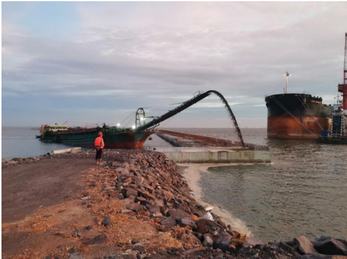
5#码头沉箱箱内回填砂
