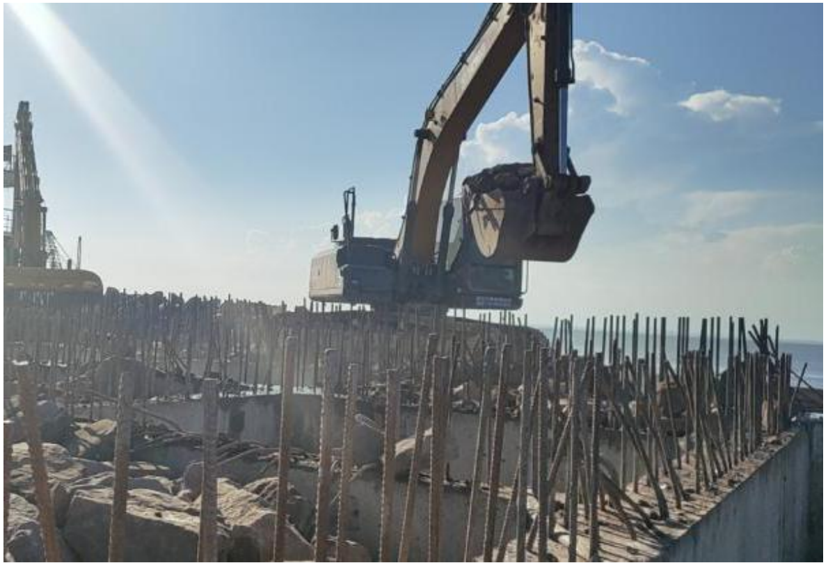
2#码头沉箱滑道处箱内回填
